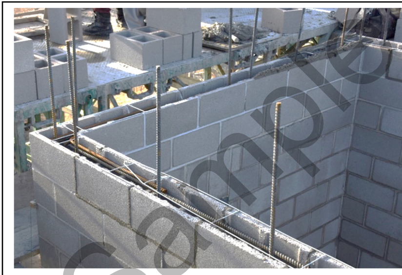
Figure 1.1 Typical Reinforced Masonry Construction
