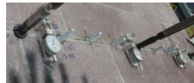
testing in cracked masonry
