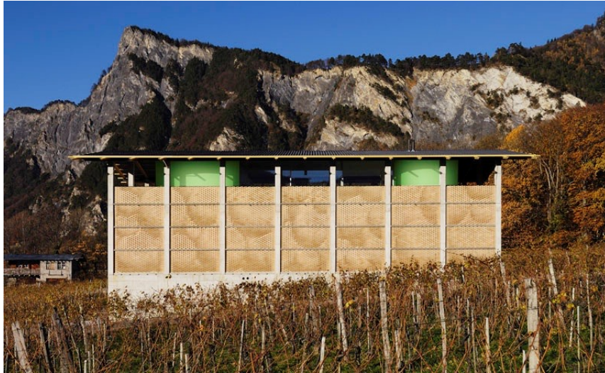
Gantenbein Vineyard Facade Beath & Deplazes Architekten ETH Collaborators: Bonwetsch and Knauss Fläsch, Switzerland 2006
