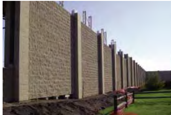
Fig. 3-23 Traffic noise from expressways can be effectively shielded by a concrete masonry wall. Photo used with permission of International Masonry Institute. ©IMI (IMG24892)
