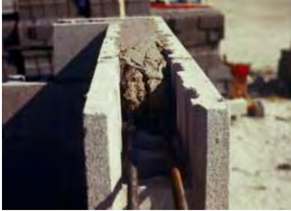
Fig. I-18 Channel bond beam. (IMG4025)
