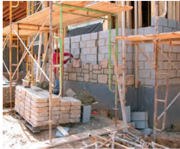
Fig. 4-8b A concrete masonry wall veneered with architectural concrete masonry units. (IMG24173)
