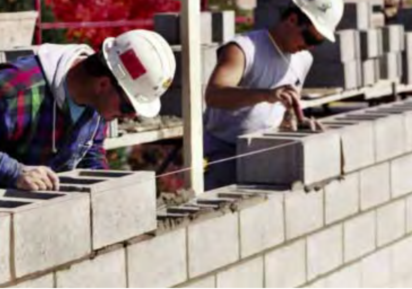
Above: Placing block into position with the aid of a stringline – see Fig. 6-26. (IMG15841) Right: Checking for plumb – see Figure 6-17. (IMG15851)
