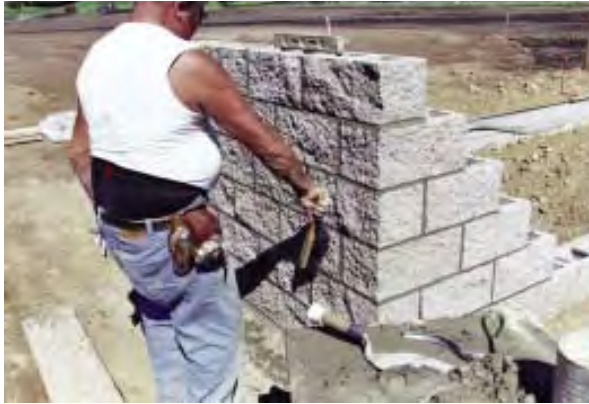
Fig. 6-59 Dressing masonry with a brush after tooling. (IMG14602)
