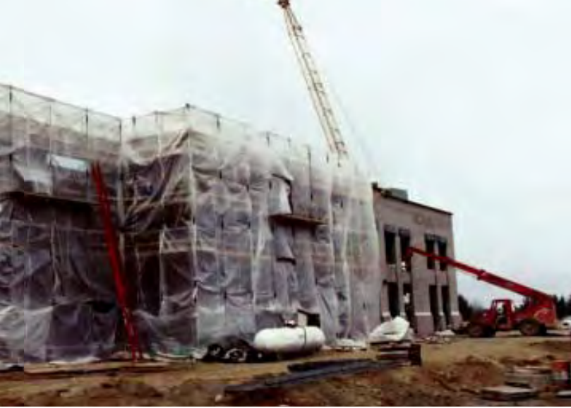
Above: Heated enclosures can extend masonry construction into colder weather — see Fig. 5-7. (IMG12504) Right: Retempering mortar is a common practice, especially during hot weather — see Fig. 2-16. (IMG13630)
