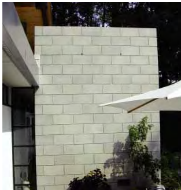
Fig. 6-61 Raked joints create stronger shadow lines and accentuate the outline of the block. (IMG17009)
