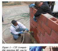
Figure 1 - CIP (compacted injection fill) can be
