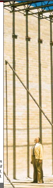
James E. Amrhein inspecting a tall masonry wall, 1998.
